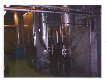
Heat recovery from humid air to water
